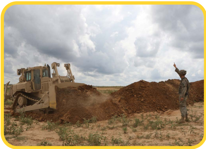
Sgt. Matthew Fuller, an equipment operator with the 1192nd Engineer Company, guides another operator during a berm emplacement for field artillery equipment during rotation 15-10 at the Joint Readiness Training Center, Camp Polk, La.
